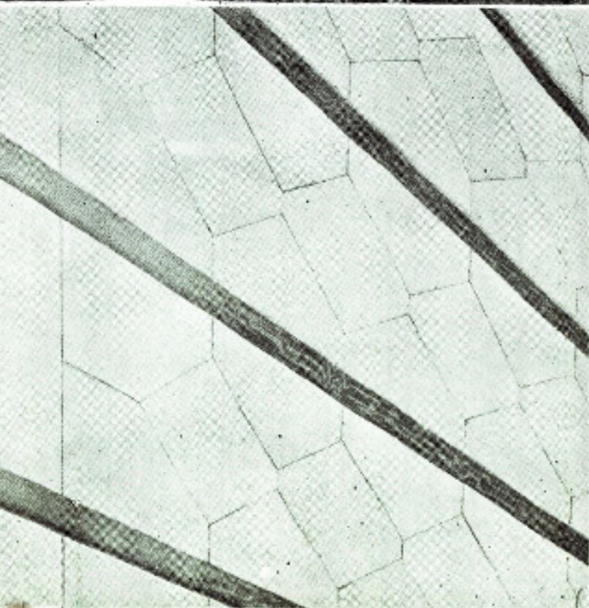
TYPICAL PATTERN OF MASONRY CLADDING ARRANGED ON STRUCTURAL PROGRESSION
